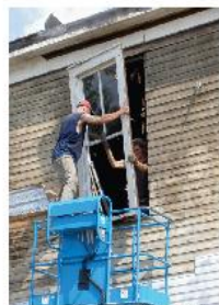
deconstruction of the existing buildings
